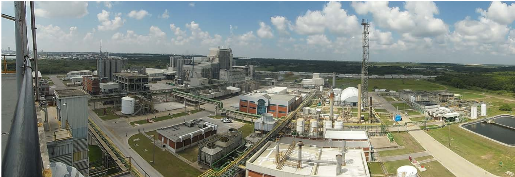
INEOS Styrolution production site in Altamira, Mexico
