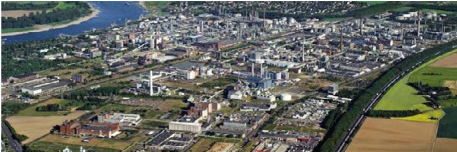
INEOS Styrolution production site in Cologne, Germany
