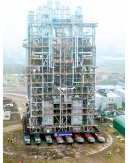
The furnaces were transported to the site using self-propelled modular transporters
