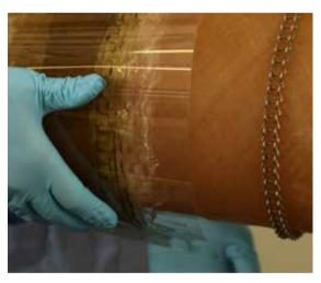
Gently press the weld strip around the surface of the pipe joint until the ends overlap; lightly press out the air bubbles with gloved hands
