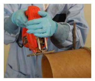
Firmly support pipe sections; square the ends to be welded using a saber saw
