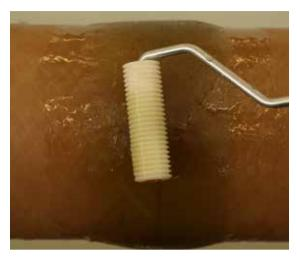
Roll out the strapping; smooth and blend the edges into the pipe surface
