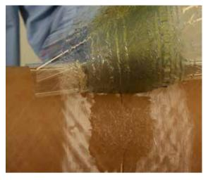
Carefully center the weld strip on the pipe joint and wrap the strip around the joint
