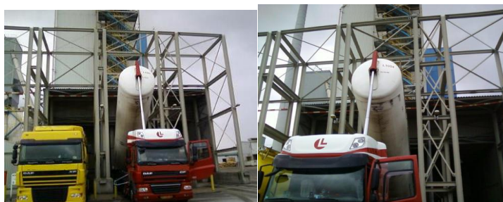
Mechanical structure to protect people/ equipment/ vehicles in the event of a silo truck falling over
