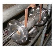
Mounting position of fitting piece on the tank near manhole:
