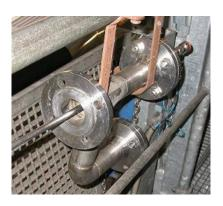
fitting piece DN 80 for venting and overfill protection:
