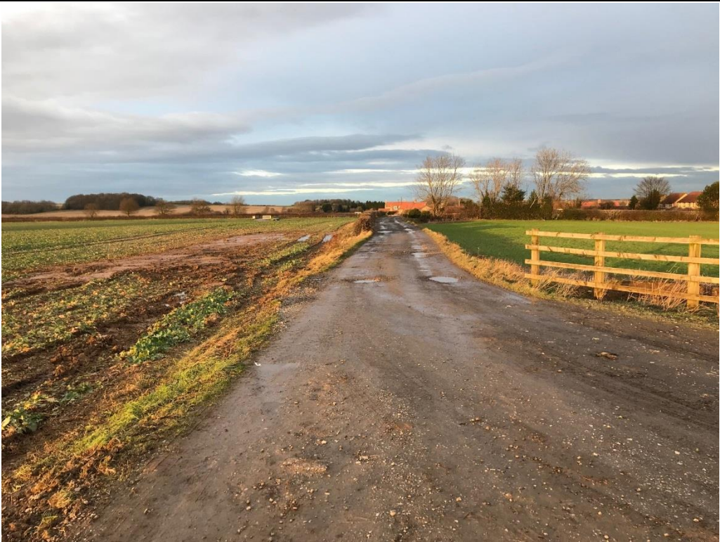
Figure.3 Access Route Looking North Towards Dinnington Road
