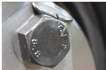
Bolt with locking plate
