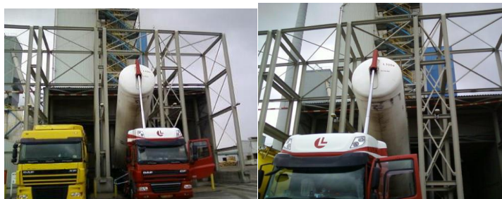
Mechanical structure to protect people/ equipment/ vehicles in the event of a silo truck falling over
