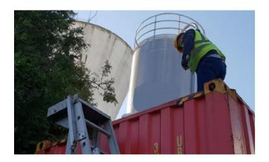
STOP climbing on top of a truck or container without the adequate protection
